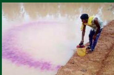
Potassium Permanganate (KmNo4) and Lime Treatment in Amrit Sarowar at Village Kartali
